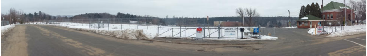
Figure 6: Panorama of the Existing Condition of the Former Mill Site
